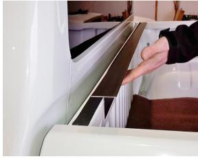
2.1) Fit the side of the "T" section extrusion with the silicon on it, down to the front of the tub as shown on the inside, with the longest leg down.
