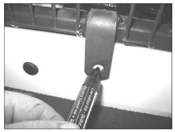
11. Mark hole centres through bottom brackets onto panel behind.
