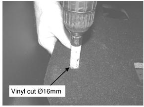
33. Using a Ø16mm vinyl cutter or wad punch cut through the floor covering at each of the marked locations.
