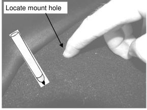
32. Locate the M10 centre holes of floor mounts, under floor covering. Mark centre point on covering with a white marker.
